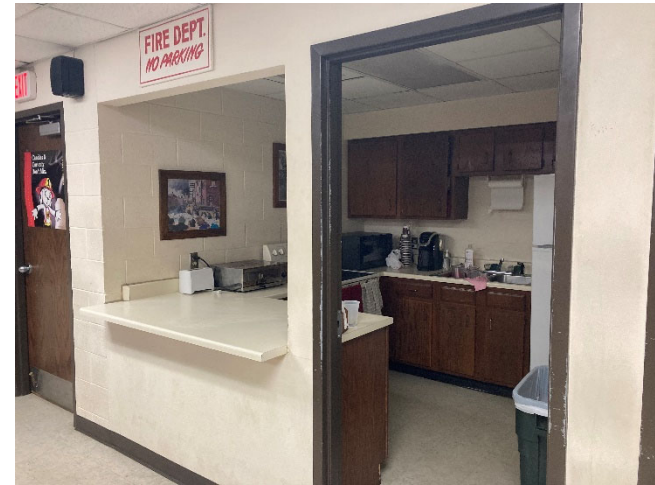
Photo 1 – Non-ADA compliant kitchen with residential grade cabinets and counter tops.
