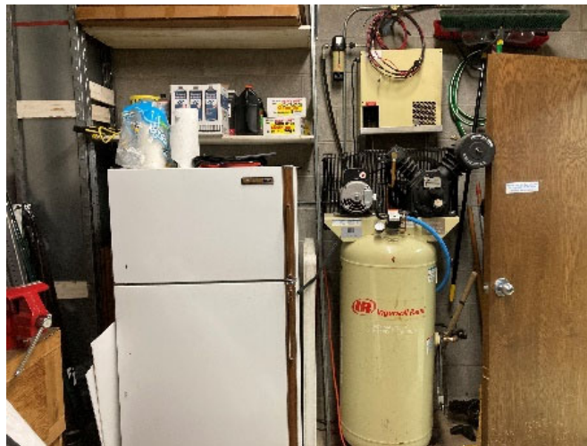
Photo 7 – The truck air compressor is in the same room as the gear laundry, computer server, and spare gear storage.
