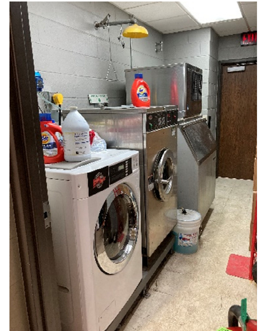
Photo 8 – Cramped conditions in the gear laundry room and non-functional emergency shower.
