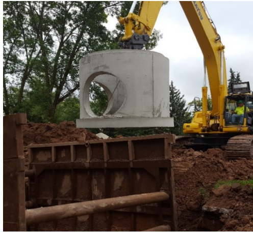
Storm manhole installation for Downtown Storm Sewer Project
