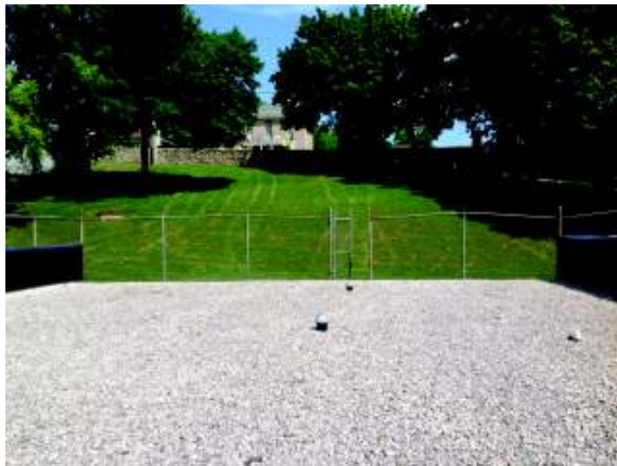
Facing North Ballasted EPDM
