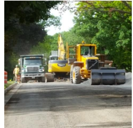
Utility Construction begins on Hayes Street.
